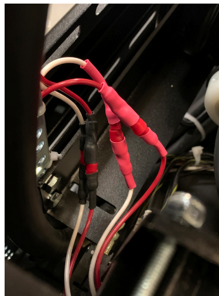
Figure 2.10 – Fan panel connections
