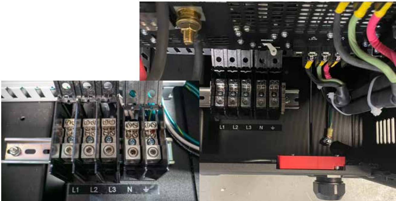
Figure 2.7 – Wiring the AC distribution block
